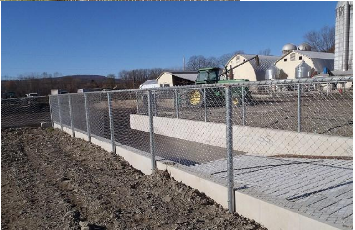
Right: Manure Storage Pit after the installation of the ramp.
