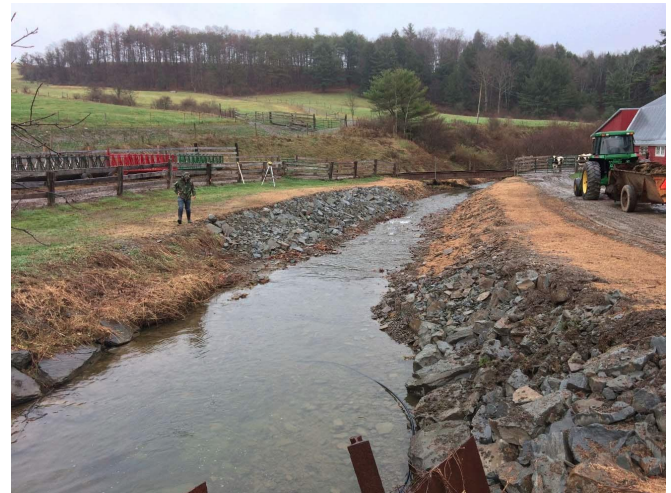
Doolittle Creek Project: photo right (230 ft. of rip rap and two stream bars installed).
