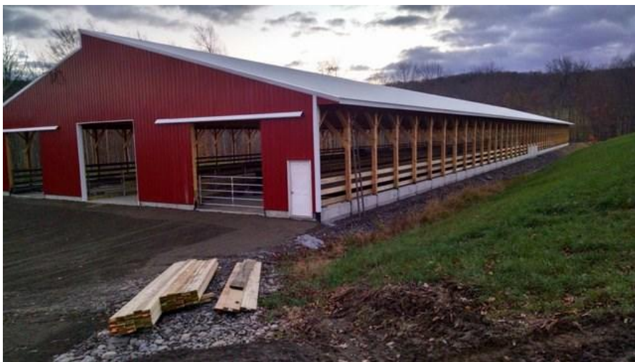
Left: Completed Covered Barnyard in Town of Newark Valley
