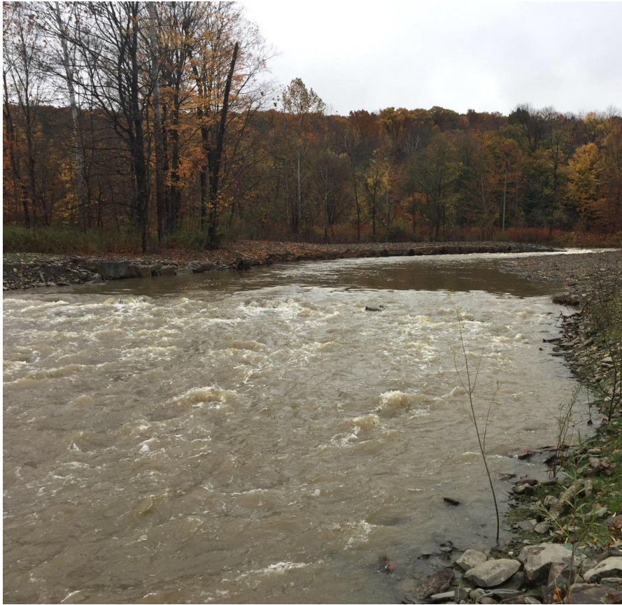
Photo Above: Apalachin Creek Stream Rehabilitation Project.
