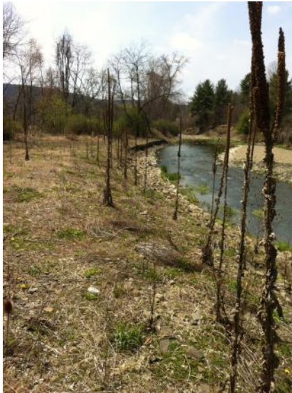
Pipe Creek: Top photos Before and after (450 ft. of rip rap installed and 4 stream bars).
