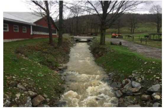
Left (Before): Undersized culvert at a farm crossing in Berkshire.
