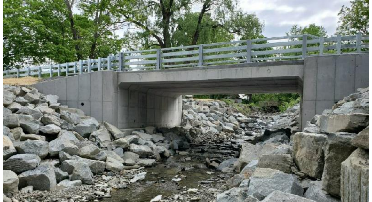
(Gaylord Stream Crossing Replacement Project, Owego, NY)
