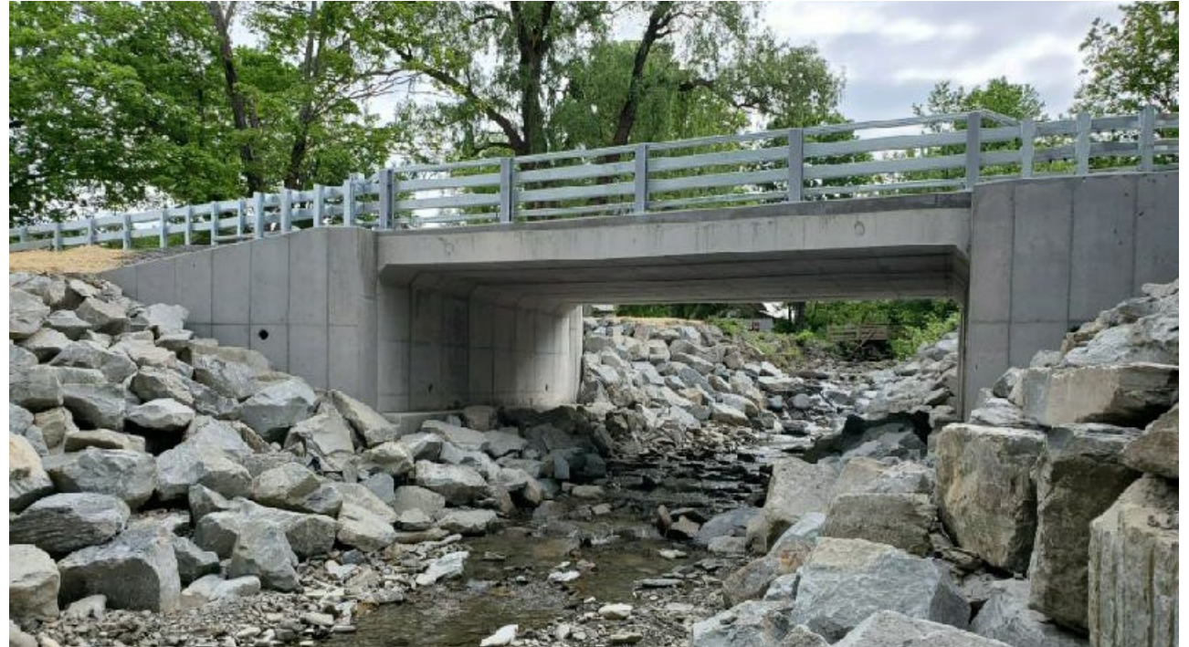
(Gaylord Stream Crossing Replacement Project, Owego, NY)
