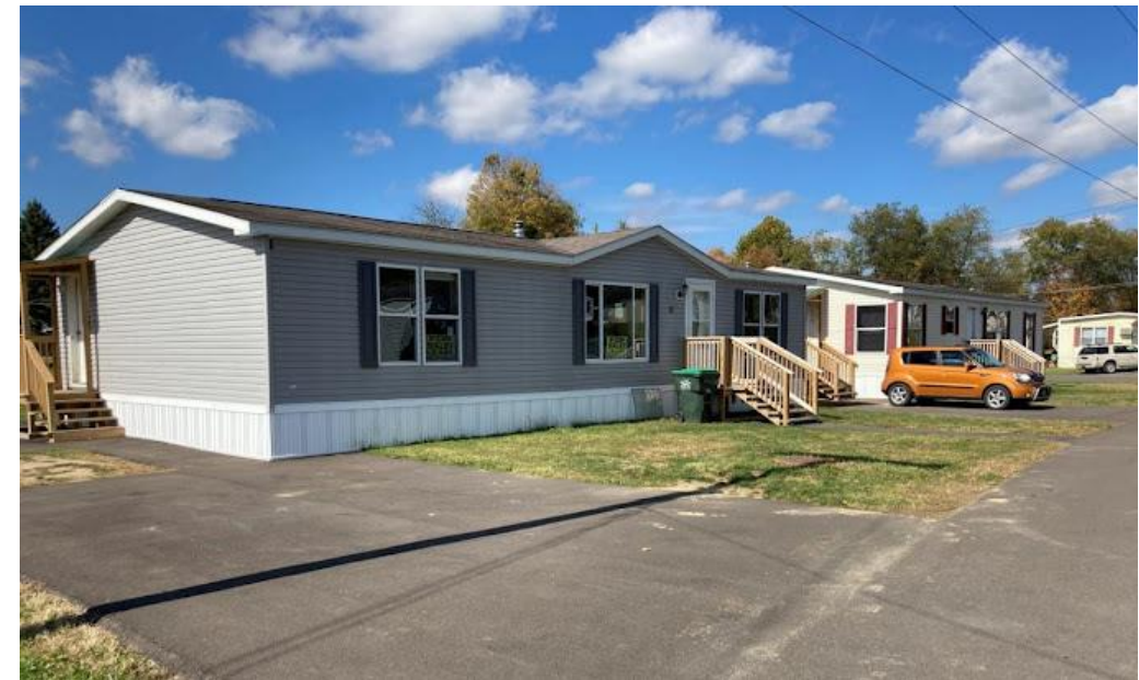
Owego Heights Mobile Home Park
